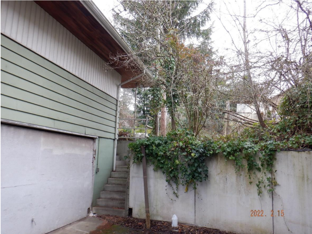
Trees #890 and #891 close to existing house
